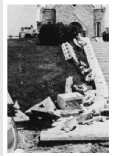
Before. Rails destroyed by a tornado.
